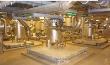
The Management Team researched filtration options available and determined that the Harmsco<sup>®</sup> Hurricane<sup>®</sup> Filtration System would meet or exceed their requirements. Because of their compact design, Eight Harmsco<sup>®</sup> Hurricane<sup>®</sup> HUR 8 X 170FL filters were able to easily fit into the existing equipment room layout.
