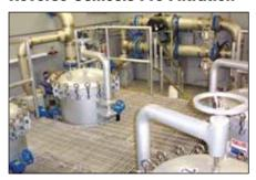
Four SB Hurricane® Swing Bolt housings were installed in parallel as pre-RO filtration using 5-micron cartridges flowing at 3,200 gpm.
