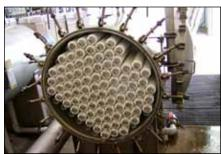
A municipal customer replaced their string wound cartridges with Harmsco® 701-5/40 pleated cartridges and experienced four times the filter life resulting in lower operation cost.
