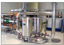
An international bottling plant installed two HIF 150FL filters in parallel with 1-micron absolute cartridges offering 2,600 sq.ft. of media, thereby maximizing their run time.
