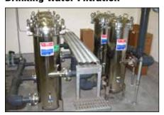
A small rural water customer installed five NSF-61 Listed HUR 1x170FL filter housings using two 5-micron NSF-61 Listed pre-filter cartridges followed by three 1-micron absolute cartridges.
