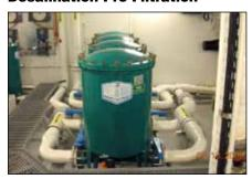
Four HIF 200FL-COAT filter housings were installed as pre-filters to a sea water RO on a cruise ship. These housings have been successfully running for the past seven years.
