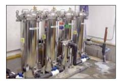
A metal finishing plant installed several Hurricane® filters with 0.35- and 1-micron cartridges to lower zinc levels in their effluent. After installation the firm was in compliance and written approval was granted.
