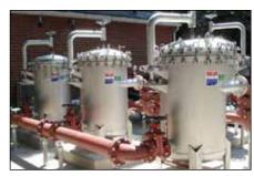
Hurricane® filters, 20- and 5-micron sediment cartridges (for pre-filtration) and 1-micron absolute rated Poly-Pleat™ cartridges for cryptosporidium control. Test results show removal requirements were achieved.
